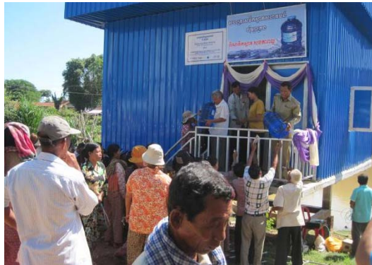
Water Treatment Plant in Cambodia set up by Lien Aid
