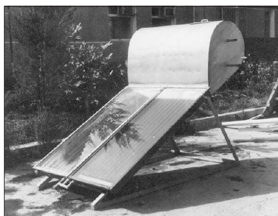
3.11. Solar water heating installation
