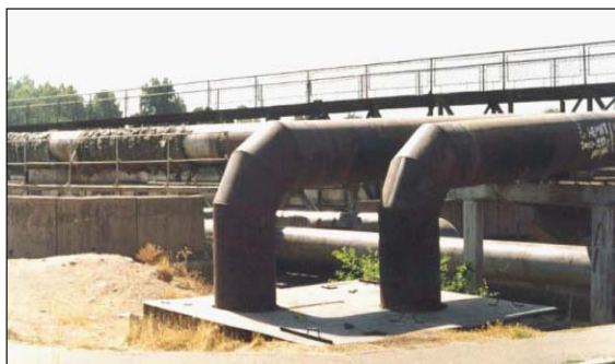
3.4. Heat distribution network in Dushanbe
