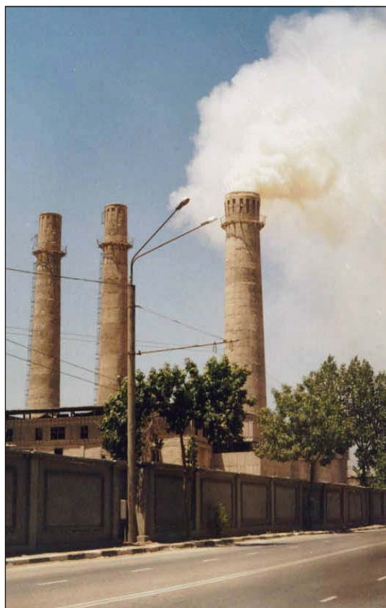
3.16. Tajik Cement Plant
