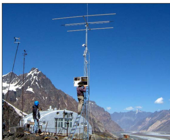
7.3. AWS mounting at the Academician Gorbunov Meteorological Observatory, Fedchenko Glacier
