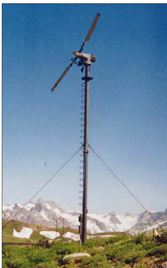
3.12. Wind power station on the Anzob pass
