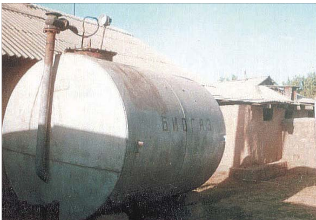
3.13. Biogas generator in rural area
