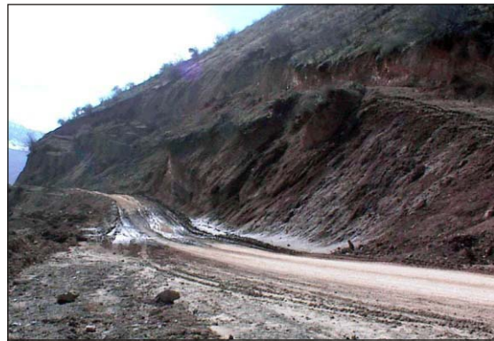
4.3. Destruction of road by natural disasters in Anzob pass
