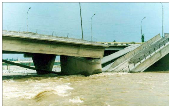
4.7. Bridge destroyed by a mudflow in the vicinity of Dushanbe
