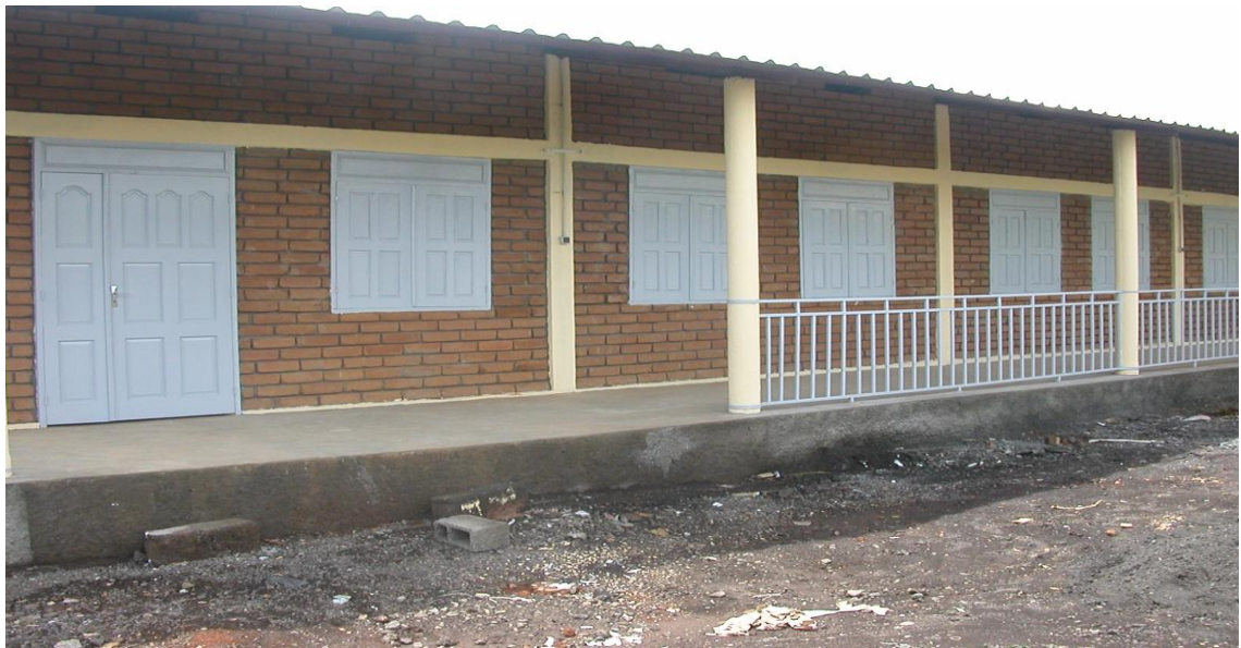
House made of bricks consolidated (case study)
