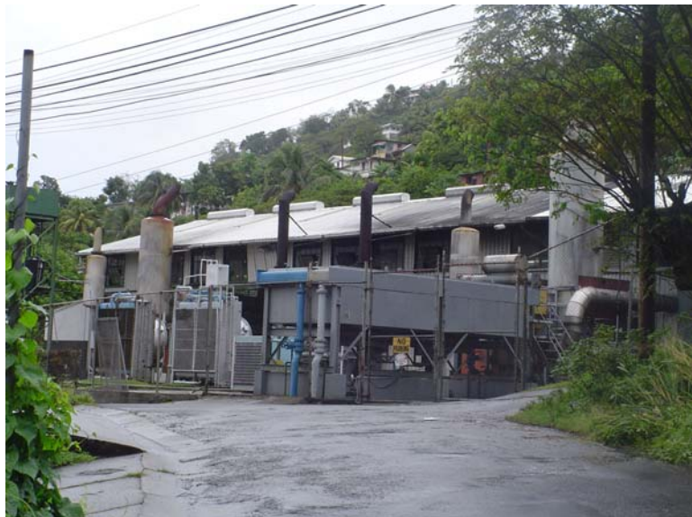
Photo 5.2 – DOMLEC Power Plant at Fond Cole
