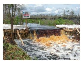
Figure A-2 Water management technology: comb structures applied to HTI drainage channel at Kampar Peninsula, Riau (left) and Tabat (right) applied to agriculture land rehabilitation in central Kalimantan (Hooijer at al, 2007)
