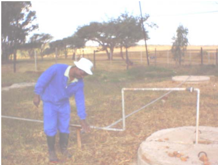
Figure 2 Biodigester at a pig-production unit.
