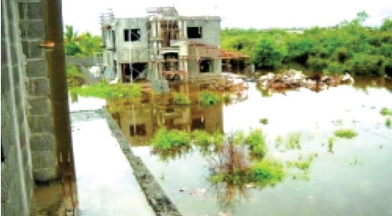
Flooding at previous wetland after having been backfilled
