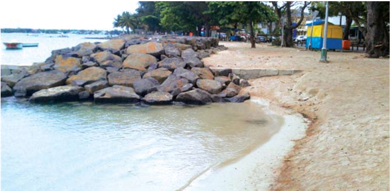
Continued beach erosion with visible escarpment at the end of rock revetment in Grand Bay
