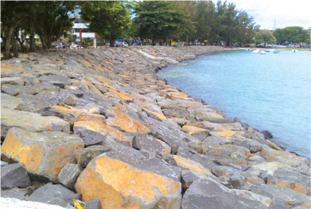
Newly installed rock revetment in Grand Bay, 2012
