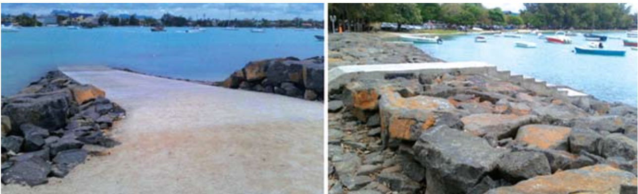
Slipway and access to the sea over the rock revetment
