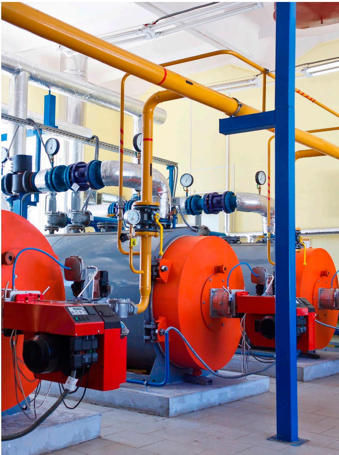
Industry boiler gas burner. Photo credit: Vladeep7/Shutterstock.com
