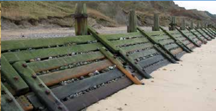
Photo: Sturdy revetments - geograph.org.uk. © Evelyn Simak, via Wikimedia Commons
