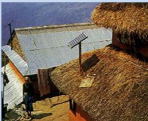
Figure 3 Solar home system
