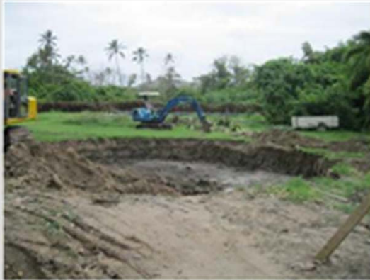
Wastewater tank excavation
