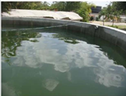
Wastewater tank in operation
