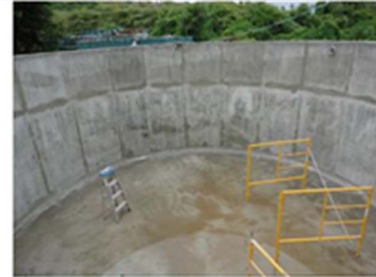
Inside waste water tank
