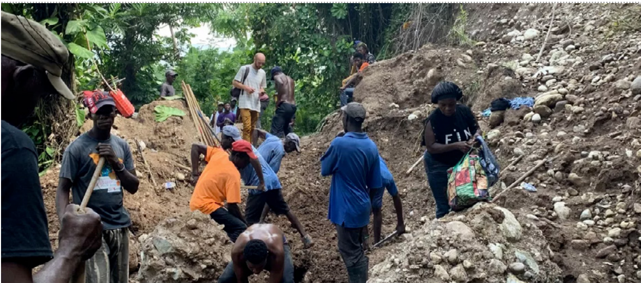
Figure 3. Recovery workers dig through debris after the earthquake of August 2021 59
