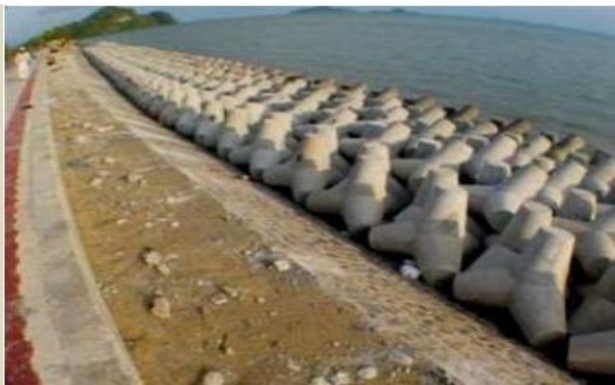
Figure 15a: Interlocking Sea Wall
