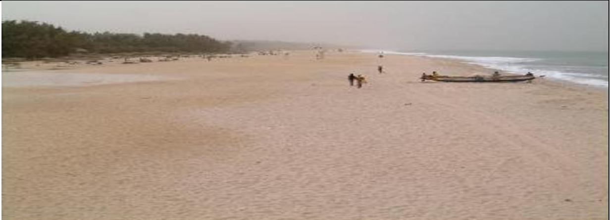
A 100-metre wide beach created after the beach nourishment of 2003 and 2004. No shoreline sand stabilization structures were added to keep the sand. What happened next? See pictures that follow
