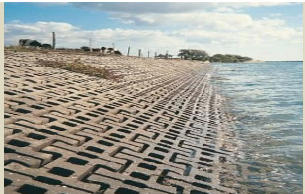
Figure 17b: Armorloc Concrete Revetment
