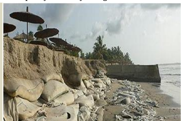
Figure 18b: An attempt to protect the Senegambia Beach Hotel against acute erosion, using sandbags
