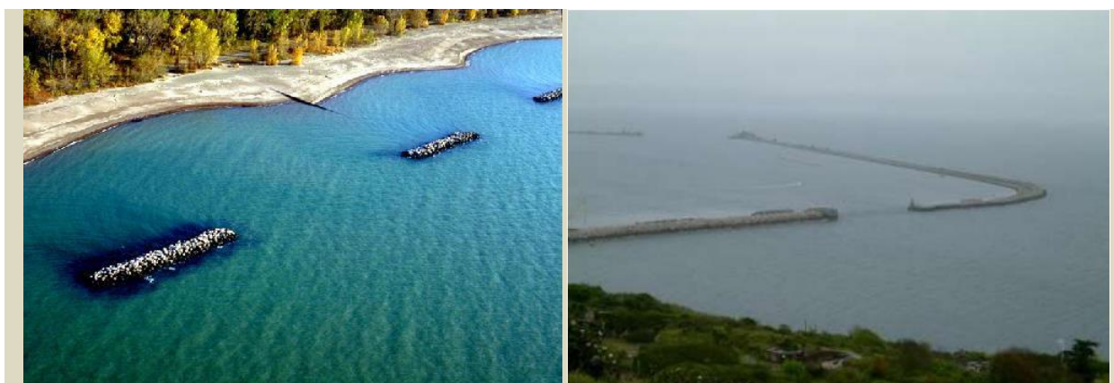
Figure 20: Examples of Breakwater Systems
