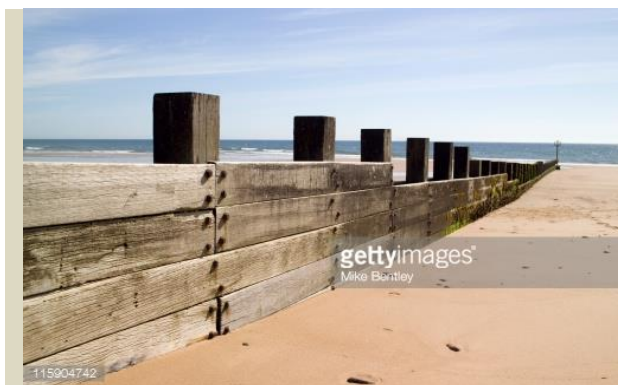
Figure 16a: Groynes made out of wooden planks
