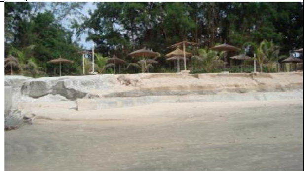
Kololi Beach Area in 2010 – 7 years after nourishment, The area is back to where it was before nourishment because there are no groins constructed to reduce the downdrift movement of the sand
