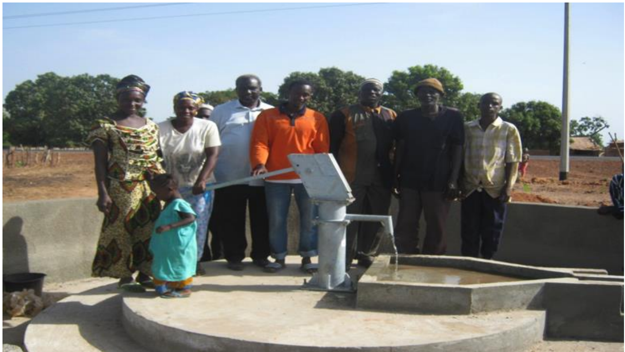
Figure 22: Hand dug well fitted with hand pump for a population of about 500 persons
