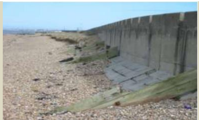
Figure 15b: Sea wall or Bulkhead similar to one at Kairaba Beach Hotel
