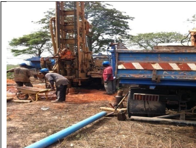
Figure 23a: Borehole drilling equipment for water supply
