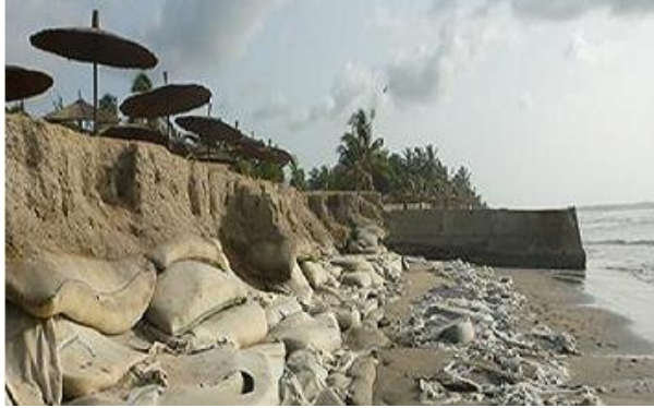
An attempt to protect the Senegambia Beach Hotel against coastal erosion before beach nourishment of 2003 2004
