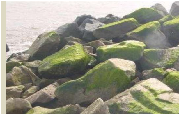
Figure 17a: Revetments constructed out of Boulders
