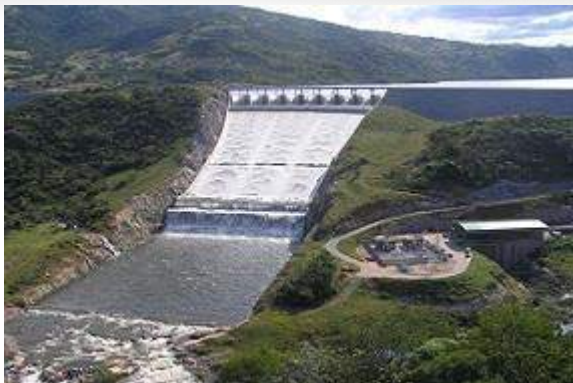
Figure 5-4: Swaziland's Maguga Dam.
