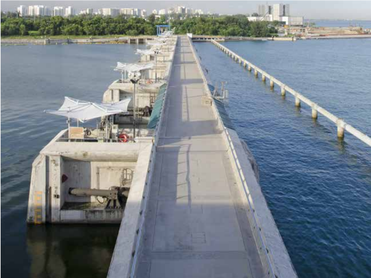
Crest gates at Marina Barrage are lowered when it rains heavily during low-tide to release excess water from the Marina Reservoir into the sea.
