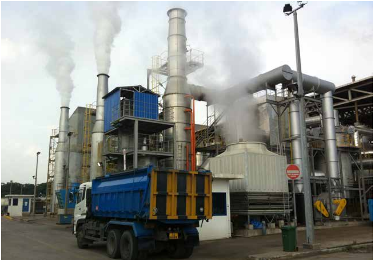
ECO-Special Waste Management (ECO-SWM) sludge incineration facility - methane emissions from sewage sludge are reduced by incinerating the sludge.
