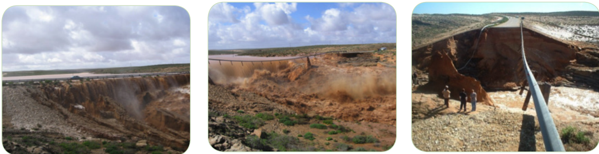
Figure 9: Flood in the Holgat River in the Northern Cape on 20 May 2006 before, during and after the bridge washed away. This area normally receives less than 200 mm of rain per year. (Photos: Johann Peyper)
