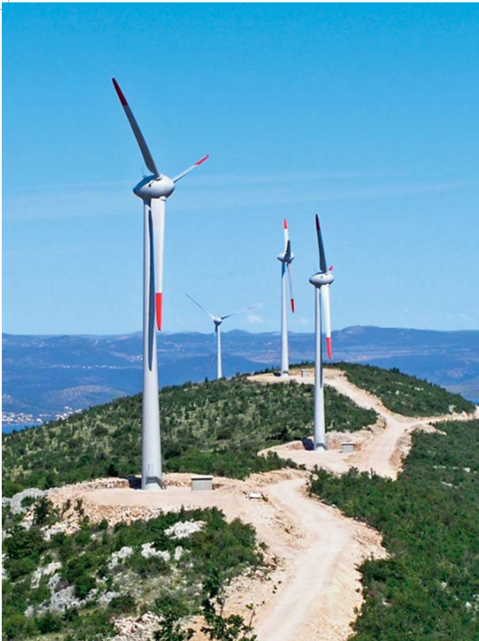
Wind power plant „Trtar – Krtolin“ in Šibenik hinterland
