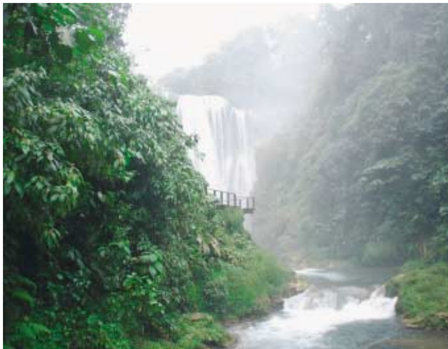
Figure 7–3 In 2005, the Rio Blanco Small Hydroelectric Project in Honduras was registered as the first Finnish Clean Development Mechanism project by the CDM Executive Board. Water flows to the turbines through an underground intake pipe; thus environmental changes in the river channel have been minimised. The waterfalls upstream of the powerplant will remain at their natural state. (Photos: Markku Nurmi).
