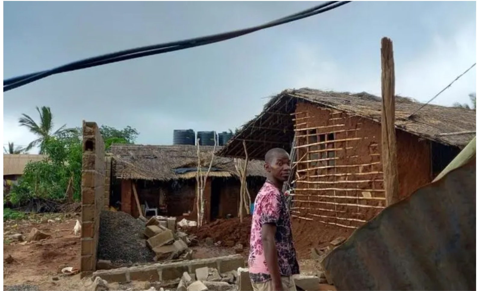
Houses damaged by Cyclone Gombe in Nampula, Mozambique. © UNHCR/Agnes Madziwa
