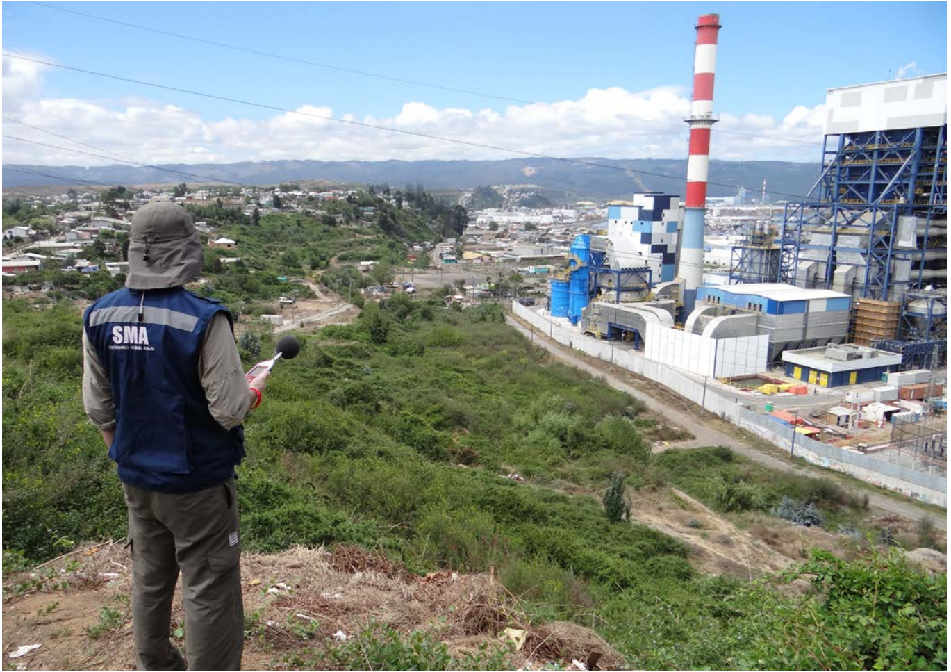
Bocamina Thermo Power Generation Plant
