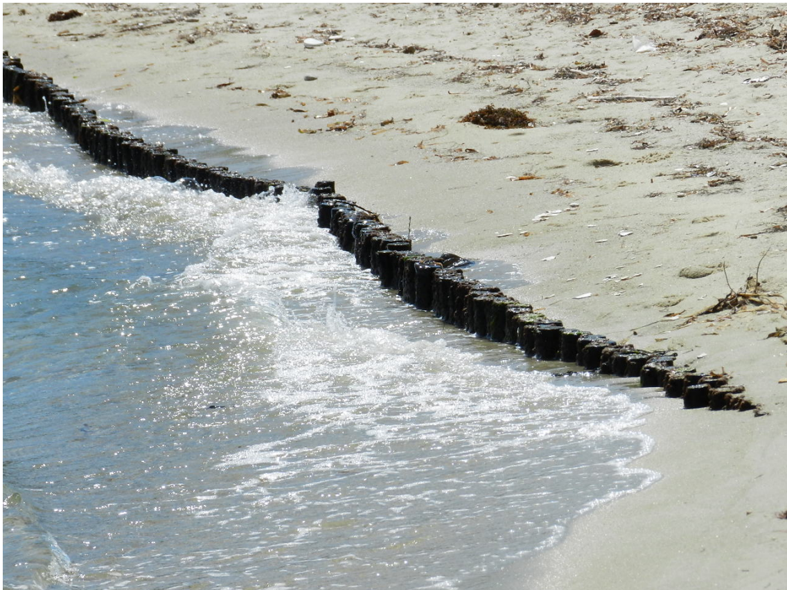
Figure 41 – Use of palmetto trunks to address beach erosion by dissipating wave action and promoting the accretion of beaches in Placencia and Monkey River
