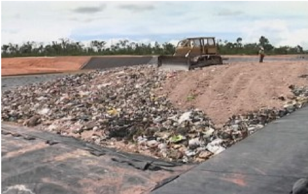
Figure 51: Sanitary Land Fill located at mile 23, Gorge Price Highway (Inaugurated 30 th July 2013) Source: Great Belize Productions Limited
