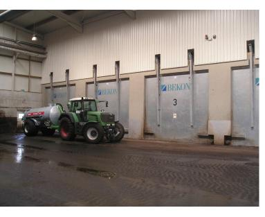
Figure 12: Batch digesters in Thun, Switzerland
