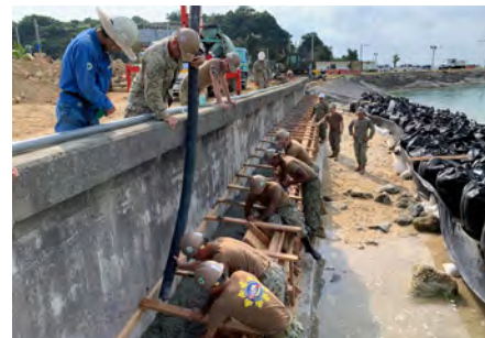
Navy Seabees deployed with Naval Mobile Construction Battalion (NMCB) 5 place concrete for the seawall project on board White Beach Naval Facility. NMCB-5 is deployed across the Indo-Pacific region conducting high-quality construction to support U.S. and partner nations to strengthen partnerships, deter aggression, and enable expeditionary logistics and naval power projection.
