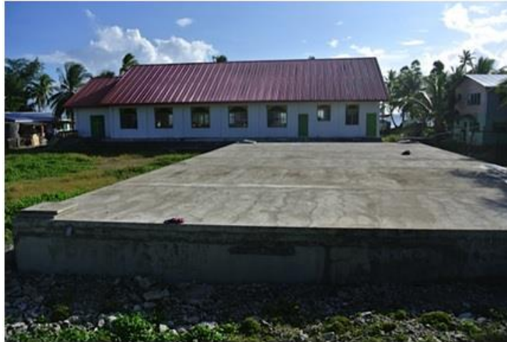
Figure 18 PACC Water Cistern installed at Lofeagai Community, Funafuti, 2012
