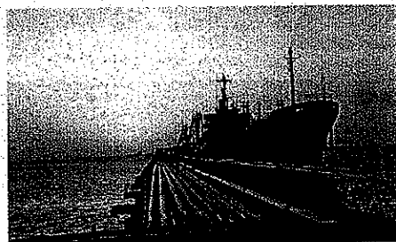
Bunkering facility, Petroleum Company of Trinidad and Tobago (Petrotrin). Courtesy Petrotrin
