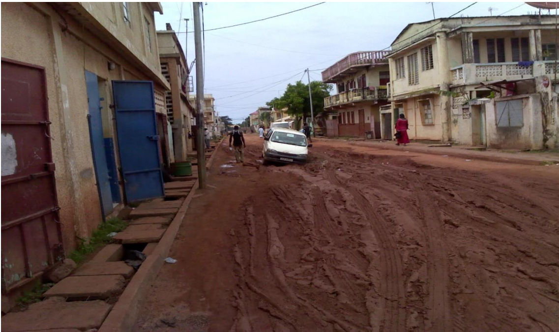
Figure 33. Poor state of unpaved roads in urban areas during the rainy season. Courtesy: Momodou Njie
