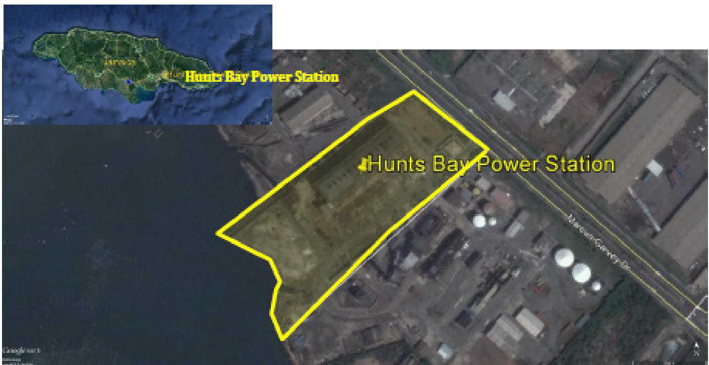
Figure 9: Hunts Bay Power Station
