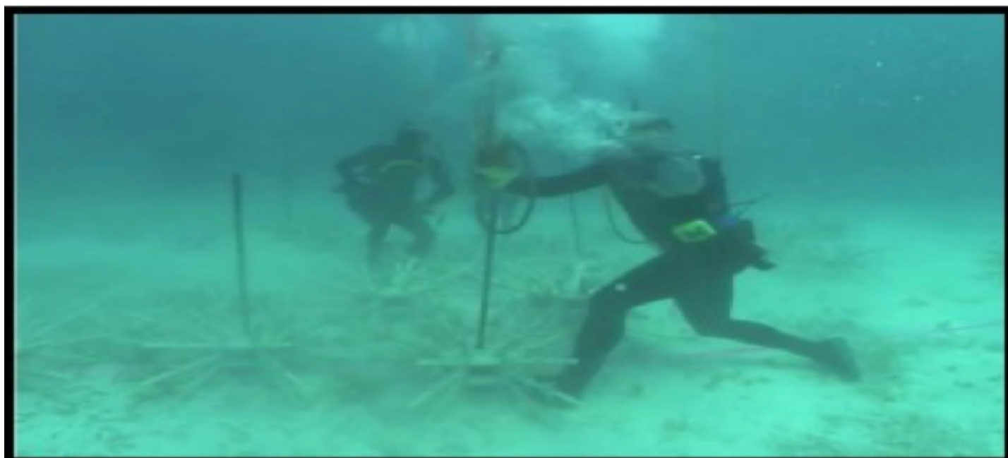
Figure 19: Installation of artificial coral reef at Bluefields Bay, Westmoreland ( https://www.ecoreefs.com/ )
