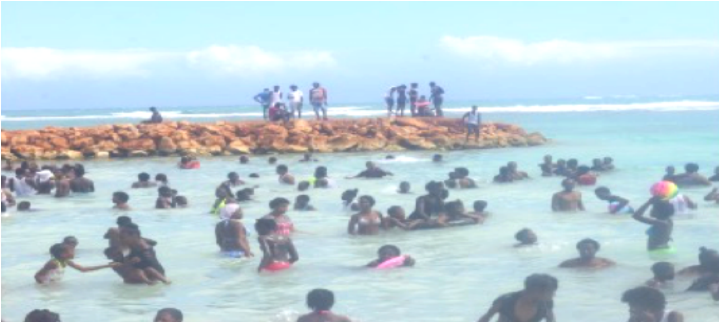
Figure 17: Groyne installed at Hellshire Beach
