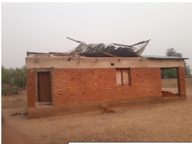
Houses will be impacted by higher wind speed. A roof blown off by strong winds (Bangula)
