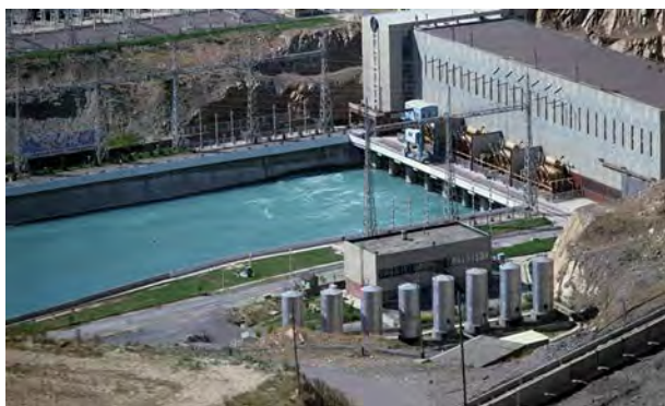
Figure 3.4 | Modernization of the third Hydroelectric Generating Unit in Charvak HPS
