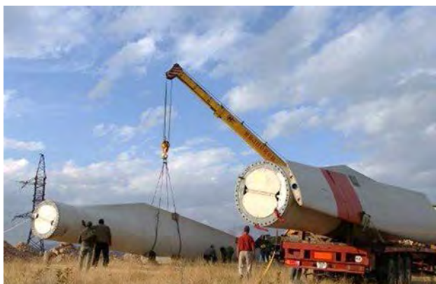
Figure 1.10 | Installation of 750KW Wind-driven Power Plant in Tashkent Province
