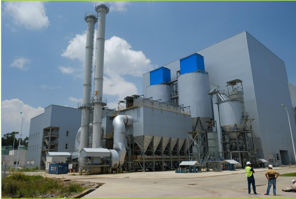
Figure 101 Reppie Waste-to-Energy facility
