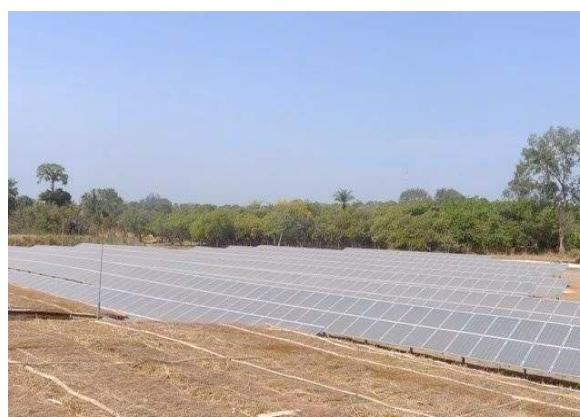
Figure 2.12 - Solar photovoltaic power plant of 314kW to produce electricity Banbadinga Sector (Banbandinga castaclar).
