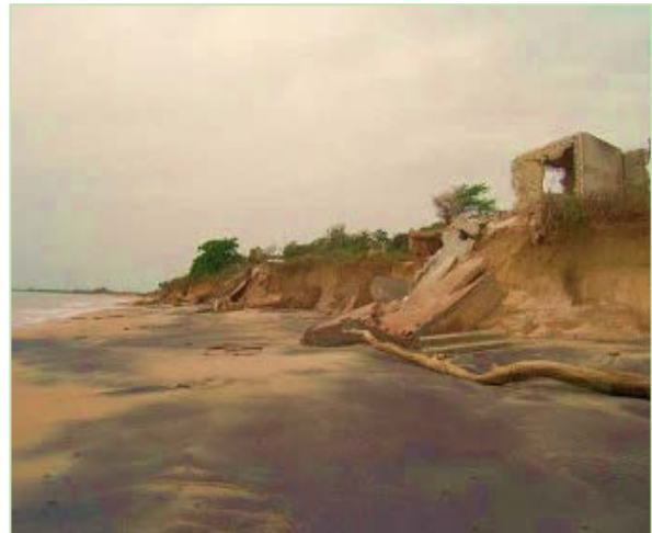
Figure 2.17 - Ruins resulting from severe coastal erosion at Varela Beach. Guinea-Bissau 76 .
