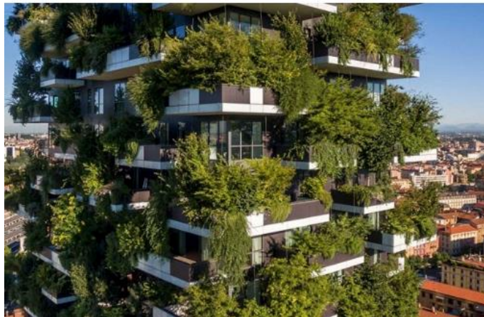
Green infrastructure – Bosco Vertical skyscraper complex in Milan
