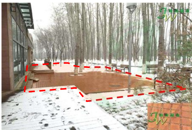
Winter: Snow Melting (Olympic Park, Beijing, China)
