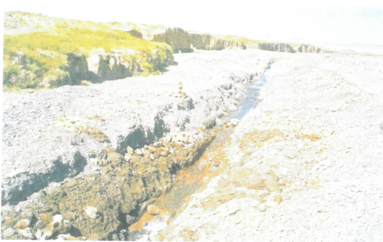
Poorly managed irrigation system in Herat
