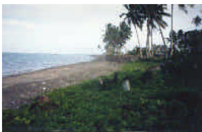
A village-based seawall project in Savai’i.
