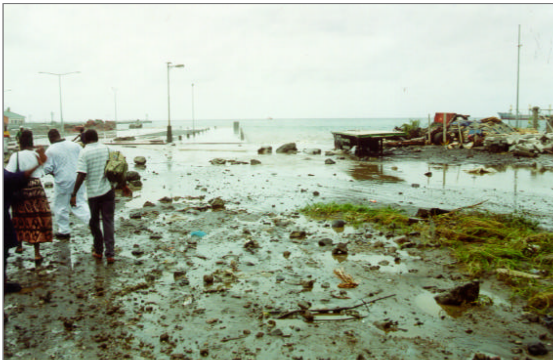
Photograph 4-4: Storm Debris near new Cruise Ship Terminal
