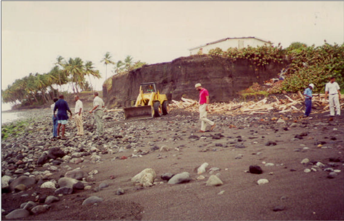
Photograph 4-1: Shoreline Erosion at Sandy Bay
