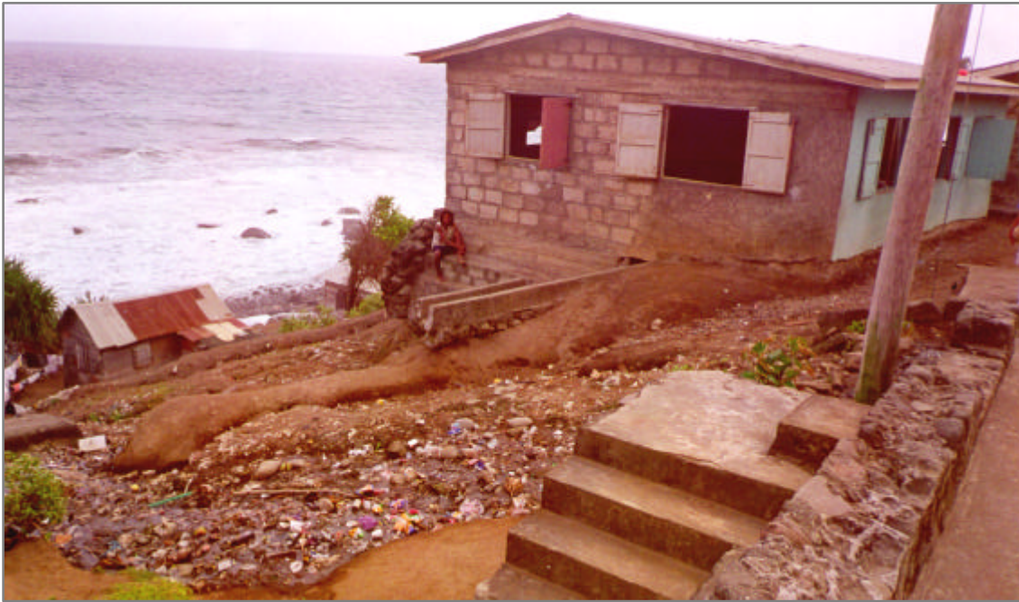
Note: Open drain with waste from the Sandy Bay Clinic -- passing outside the Sandy Bay Primary School
