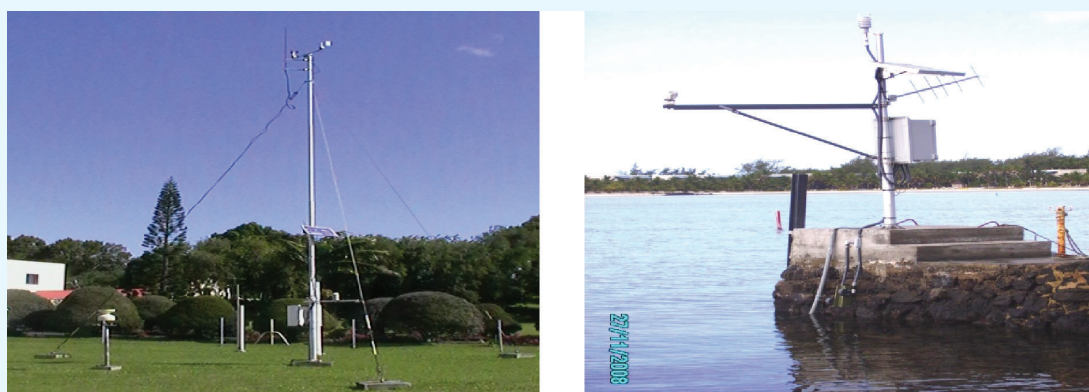
Figure 6.4 - An automatic weather station and, a tide gauge (right). (Courtesy : MMS)
