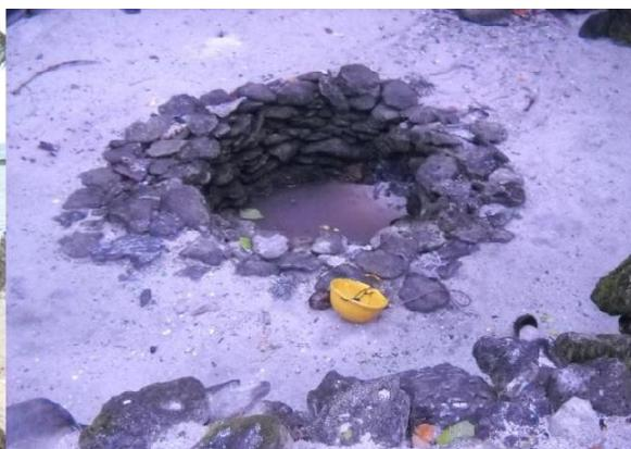
**Plate 9.** Well water exposed to salt water intrusion
