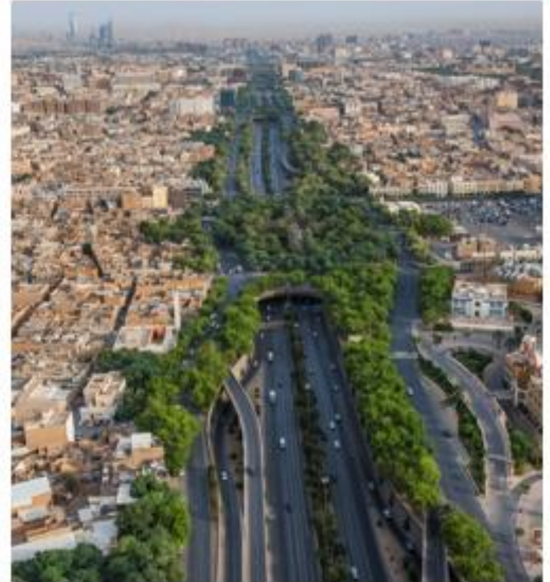
Road Greening (King Fahad Road)
