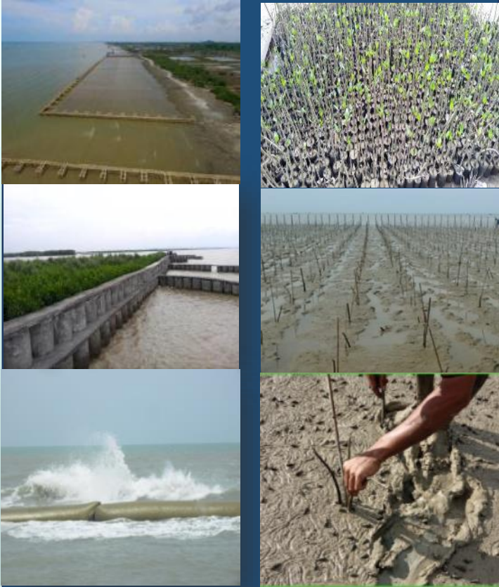
Sediment traps & mangrove rehabilitation
