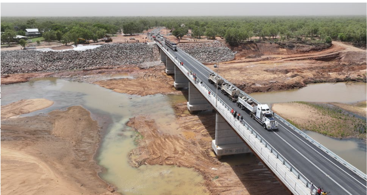
Re-connecting the Kimberley region with the re-opening of the Fitzroy River bridge. Credit: Main Roads Western Australia
