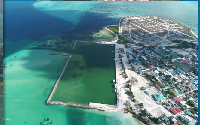
Thulhaadhoo Shore Protection and Harbour Project
