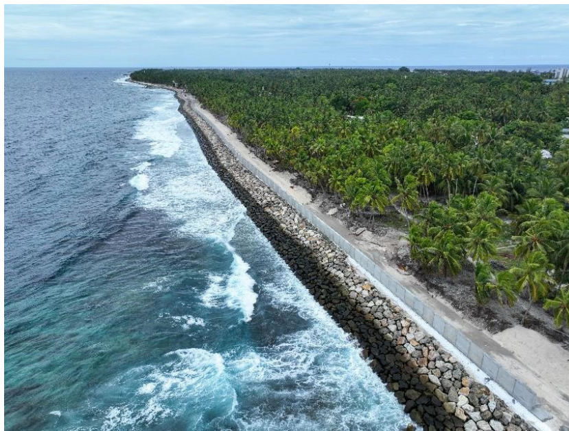
Often, hard engineered measures are seen as the only viable solution for protection from extreme conditions. Revetments in Fuvahmulah. Photo: Water Solutions
