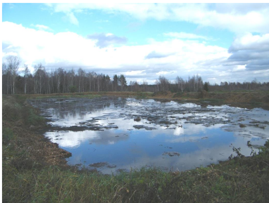
Figure 7.12 Liquid sewage sludge storage basin. Considered to be source of CH 4 emissions (deep anaerobic lagoon)
