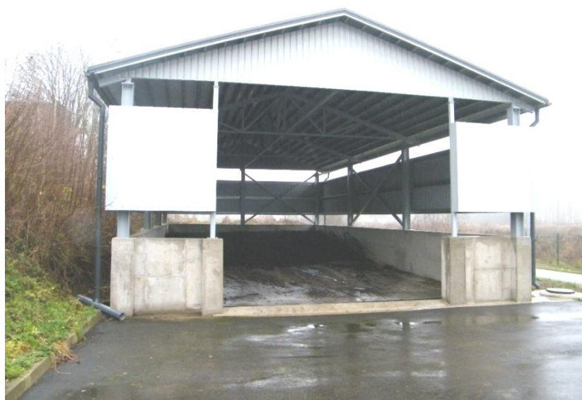
Figure 7.12 Dewatered sewage sludge storage shed. Considered to be no source of CH 4 emissions
