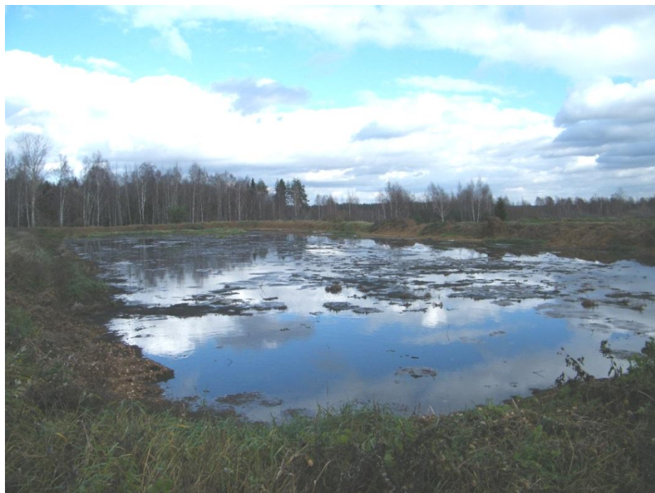
Figure 7.13 Liquid sewage sludge storage basin. Considered to be source of CH 4 emissions (deep anaerobic lagoon)
