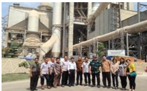
【Waste heat recovery in cement industry】 (Indonesia) 149,063tCO 2 /y. Start operation: Jun. 2018.
