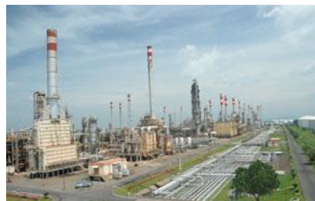
【Operation Optimization in Utility Facility】 (Indonesia) 34,956t Start operation Dec. 2017
