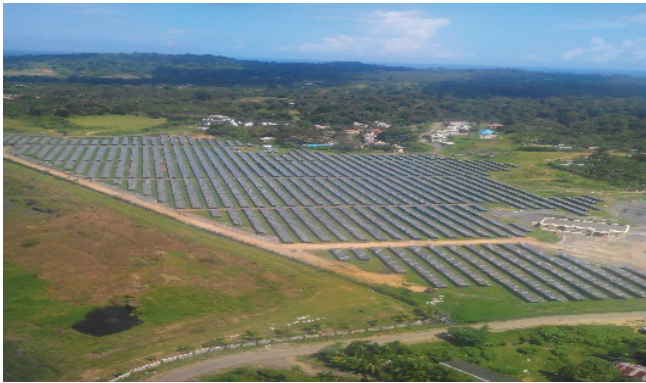
Figure 6.6: 5 MWp Solar PV Plant commissioned at Garcharma, Port Blair, Andaman & Nicobar islands
