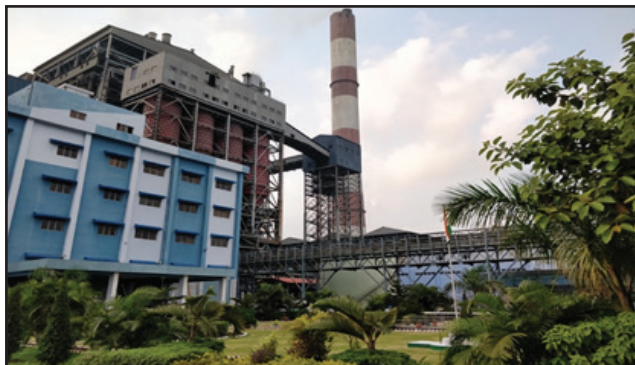
Figure 2.13: A photograph of 2 x 525 MW Coal based Thermal Power Plant in India
