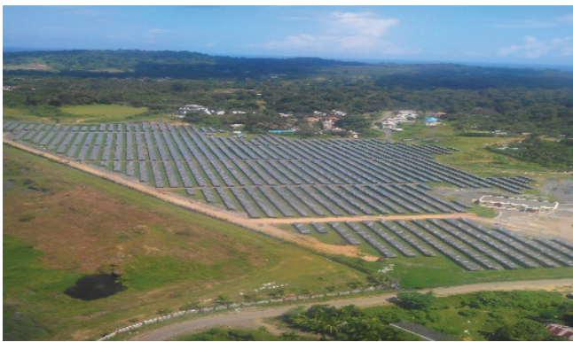
Figure 6.6: 5 MWp Solar PV Plant commissioned at Garcharma, Port Blair, Andaman & Nicobar islands
