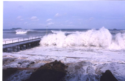
Photo 3: Hurricane Lenny Storm Surge
