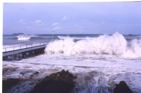
Photo 1: Hurricane Lenny Storm Surge
